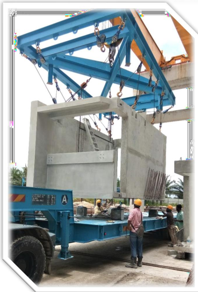
PREFABRICATED PREFINISHED VOLUMETRIC CONSTRUCTION (PPVC) AT VELOBUILD'S FACTORY, AYER HITAM, JOHOR
