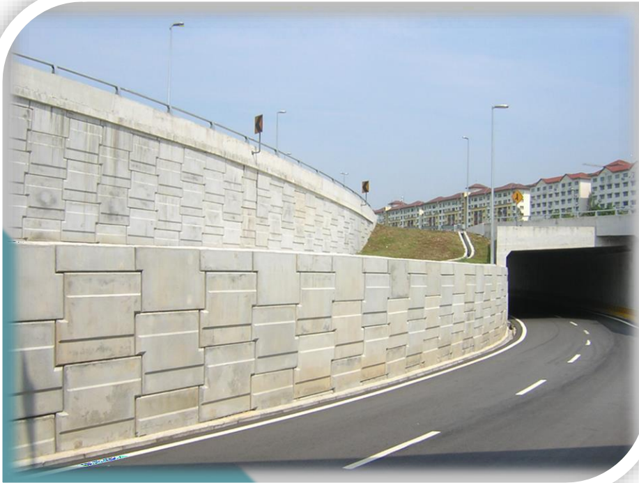
NEW PANTAI EXPRESSWAY - RE WALL AT RTM SLOPE
